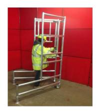
2) OPEN FRAME AND LOCK MECHANISM
